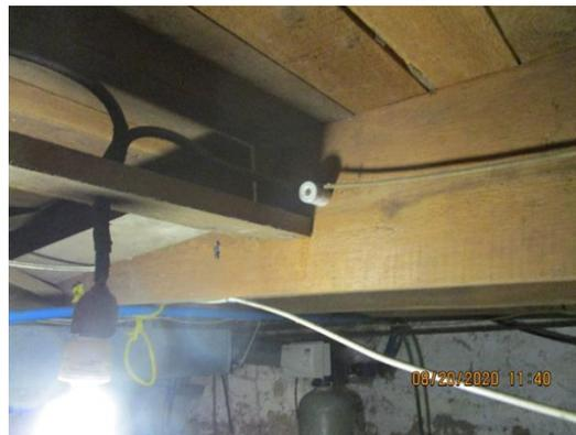
**Plate 19: Active Knob and Tube wiring feeding light**
