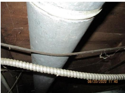
**Plate 20: Knob and Tube wiring without protect from a forced air duct**
