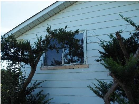
**Plate 14: Northwest window with evidence of water intrusion**
