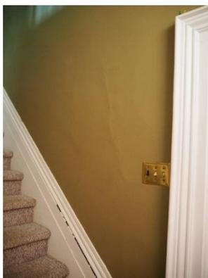
**Plate 16: Localized plaster cracks in the entrance hallway**
