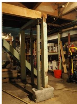
**Plate 21: Metal supports resting on concrete blocks**
