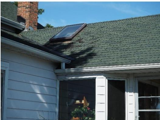
**Plate 12: Localized areas of lifting shingles**
